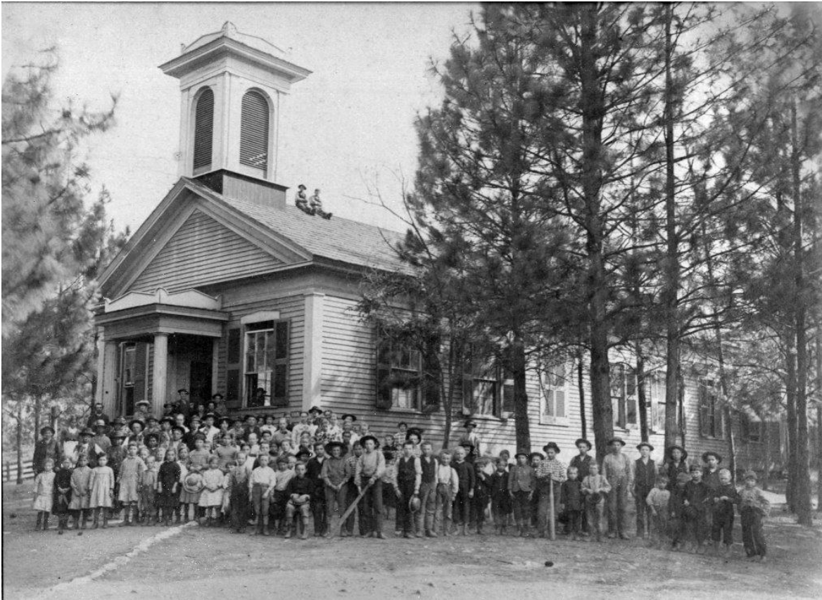
View 5: Murphy's School – see text for relationship to Douglas Flat School. Note: Building is larger and more ornate, and attention is drawn to the similar cresting on the bell tower and the porch roof. Also, the porch design is more in keeping with the Revival style.
