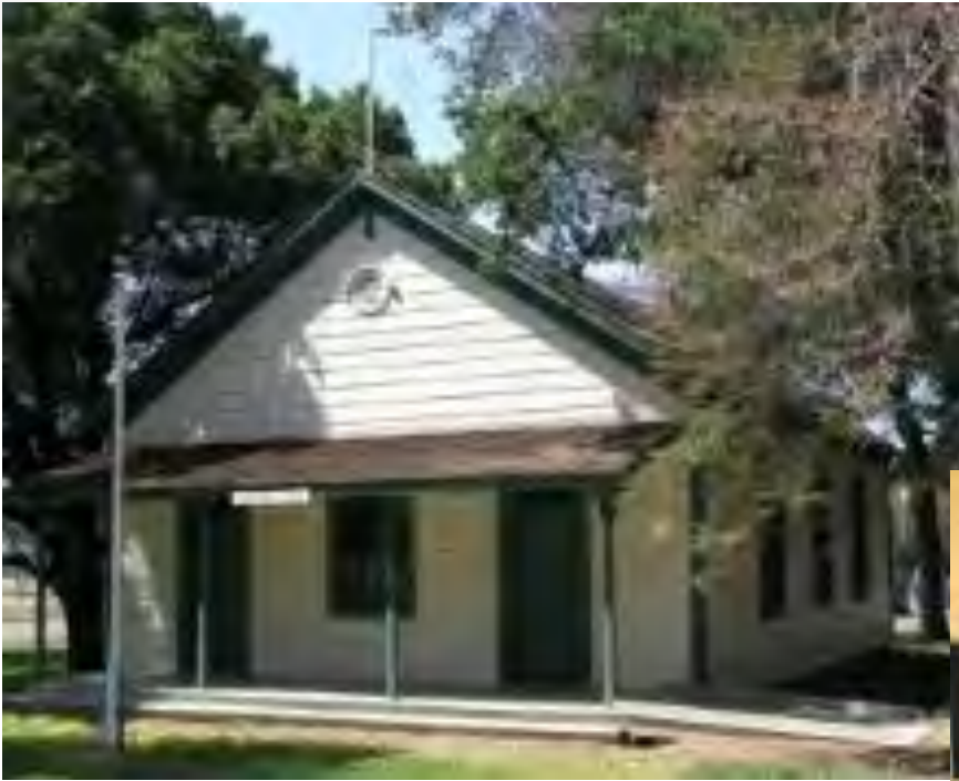
View 2: Santa Anna School, (ca. 1860s) Moved from rural San Benito County to San Jose History Museum (2002) and restored by Mineweaser & Associates, Preservation Architecture . Note: Similar, simplified Greek Revival, but separate front doors for boys & girls; new disabled access ramp.
