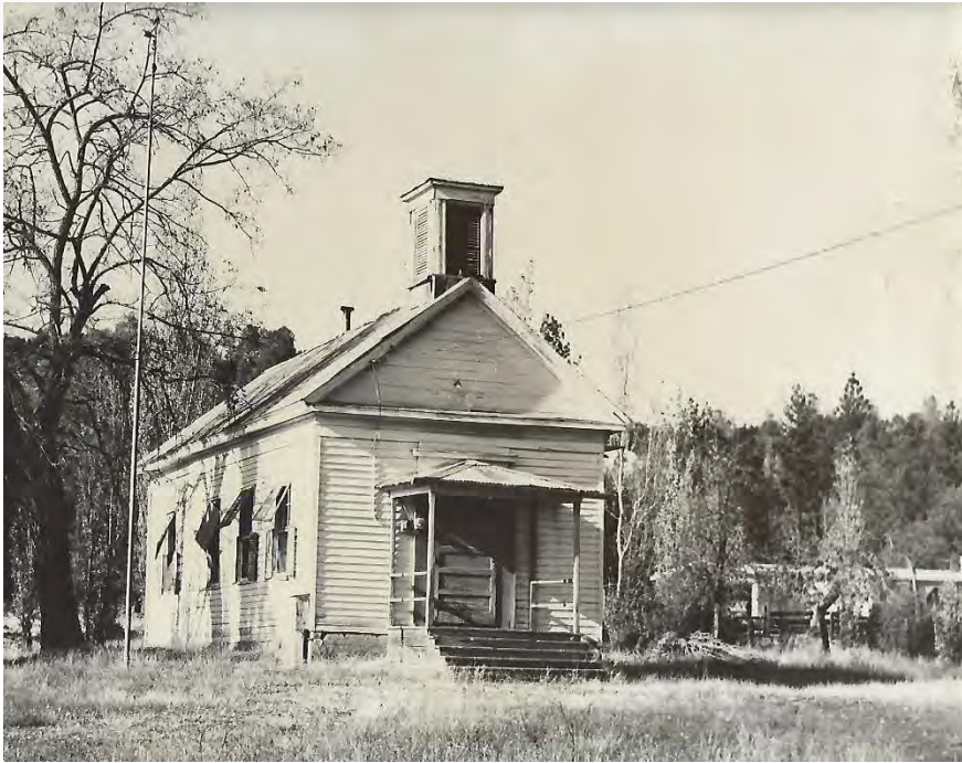
View 11a: DFS (Jan. 1971) Note single front door, lower left side at front: electric entrance, and concrete foundation distressed
