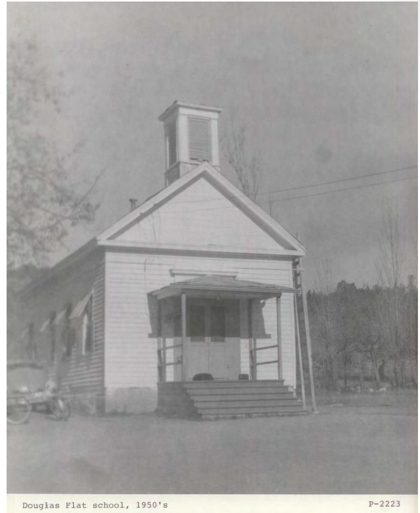
View 10: DFS (ca. 1950s) Note cresting & flag pole gone, new corrugated metal roofing likely from roof, porch modified, shutters & ladder still extant, double doors changed, concrete at parts of foundation walls (see 1925 view)
